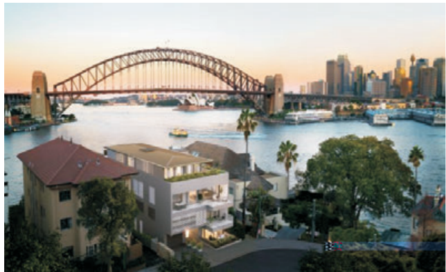
Car Lift- 3 East Crescent McMahon's Point
